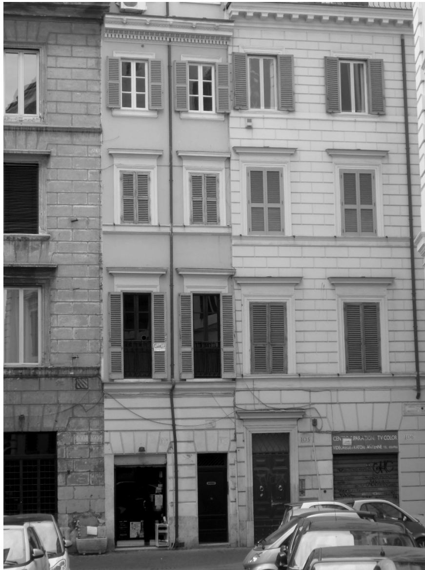
EDILIZIA (building) The type of housing unit that is the origin of much of the forming processes of European cities, developed mostly from XIII to XIV centuries, is above all the row house , a single-family building with direct access from the route that has in common with the other unities two walls.
